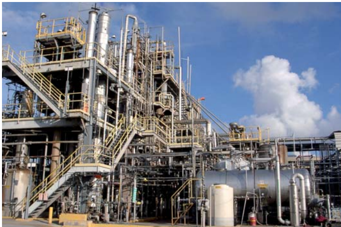
Galata Chemicals LLC production site at Taft, Louisiana, USA
